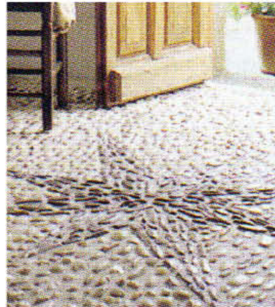
Floor designs, often with a sun or moon, are traditional and should be encouraged. The floor above is designed with local river stones and cobblestones.
