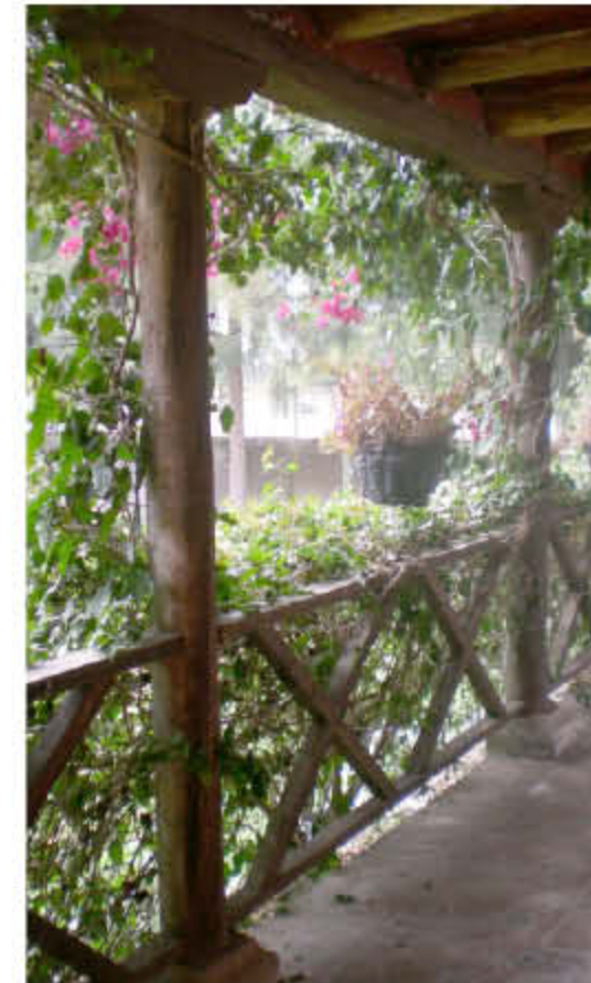
Columns should be designed in coordination with appropriate railings, trellises, and vegetation.
