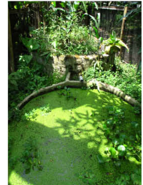
grey-water filtration tank - an aesthetic garden amenity
