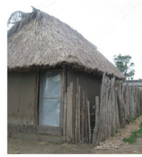
Bahareque, the lightest option, can be as thin as 10 cm.
