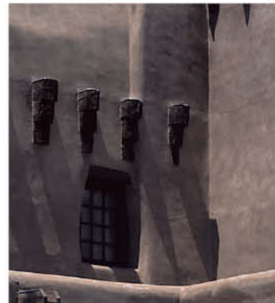
Adobe requires a minimum wall thickness of 30 cm.
