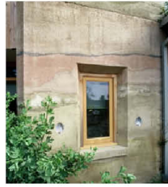
Rammed Earth varies in thickness between 75cm and 100cm.
